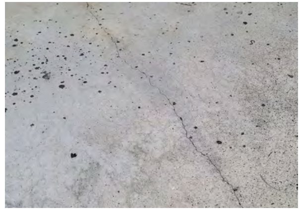
10 Cracked Concrete
