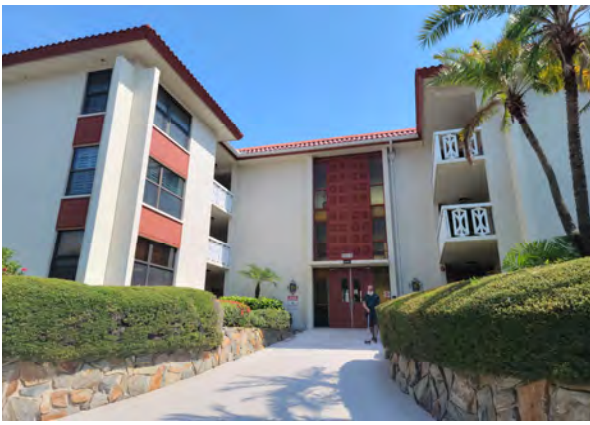
1 Front of Building
