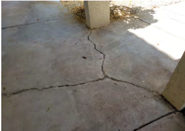
11 Cracked Concrete
