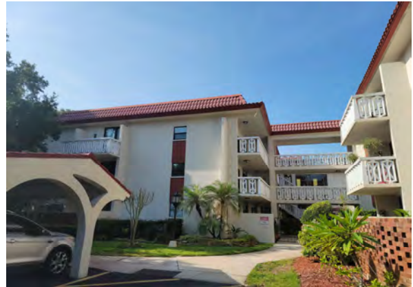
4 Left Side of Building
