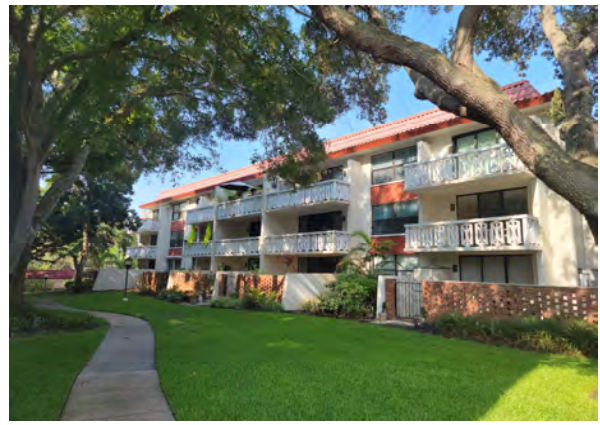
2 Right Side of Building
